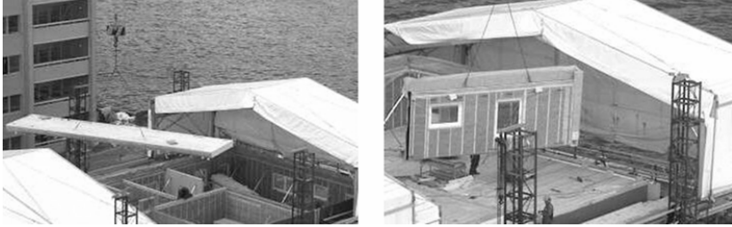
Figure 4 Assembly of floor and wall element on the construction site.
