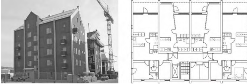
Figure 2 Left: the multi-storey timber housing project (picture by Svante Harström). Right: the basic floor plan of all houses.
